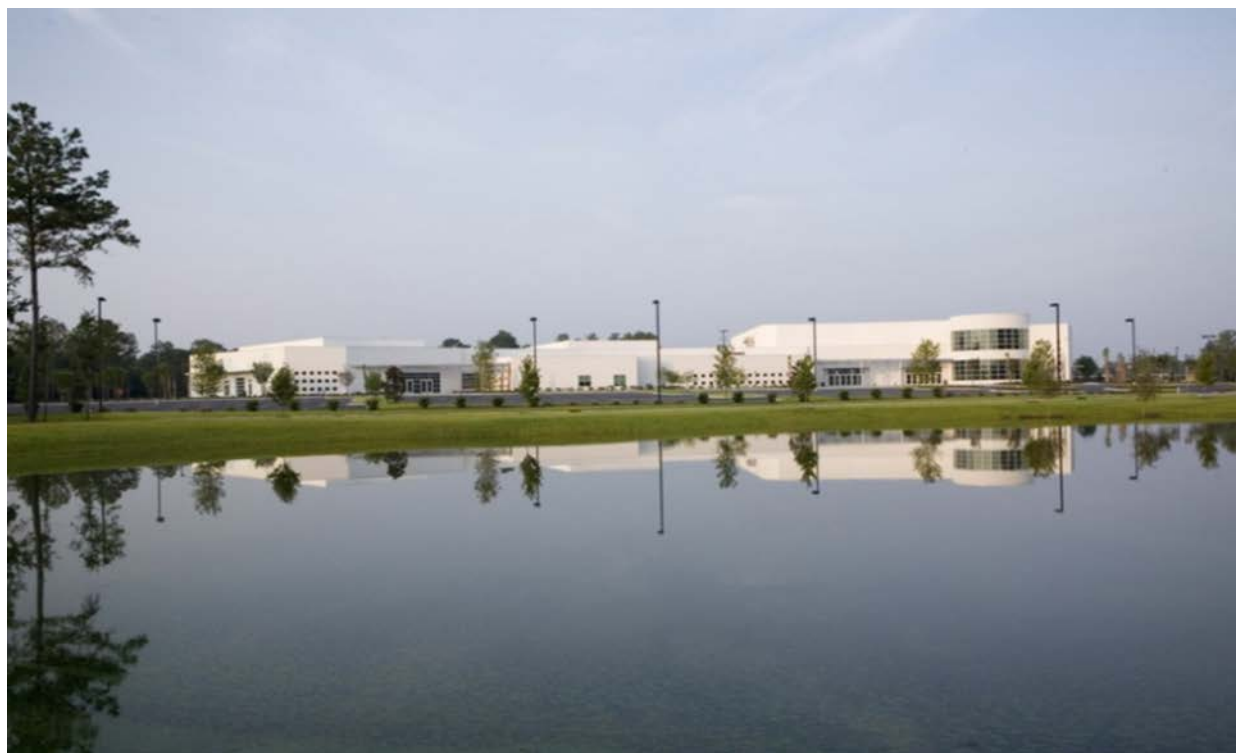
Figura 2. Instalaciones de Port City Community Church
